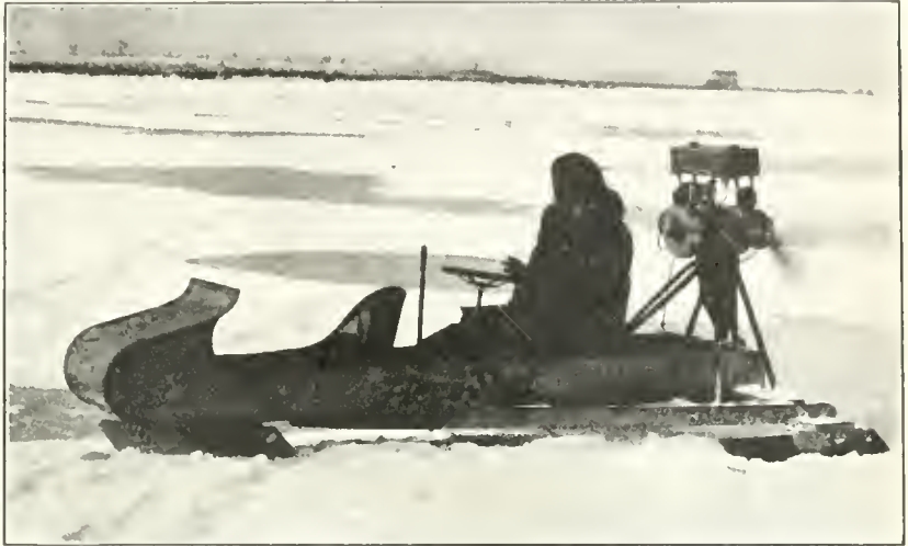
A PROPELLER-DRIVEN SLED ON THE SHREWSBURY RIVER
